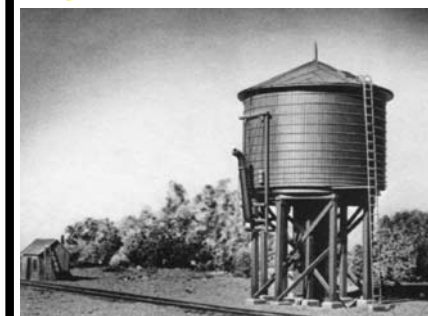
WATER TANK #A-7345
